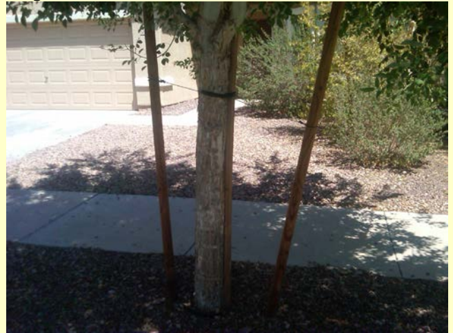
Tree stake and nursery stake left on tree for over 4 growing seasons. Support tie is girdling the trunk.
